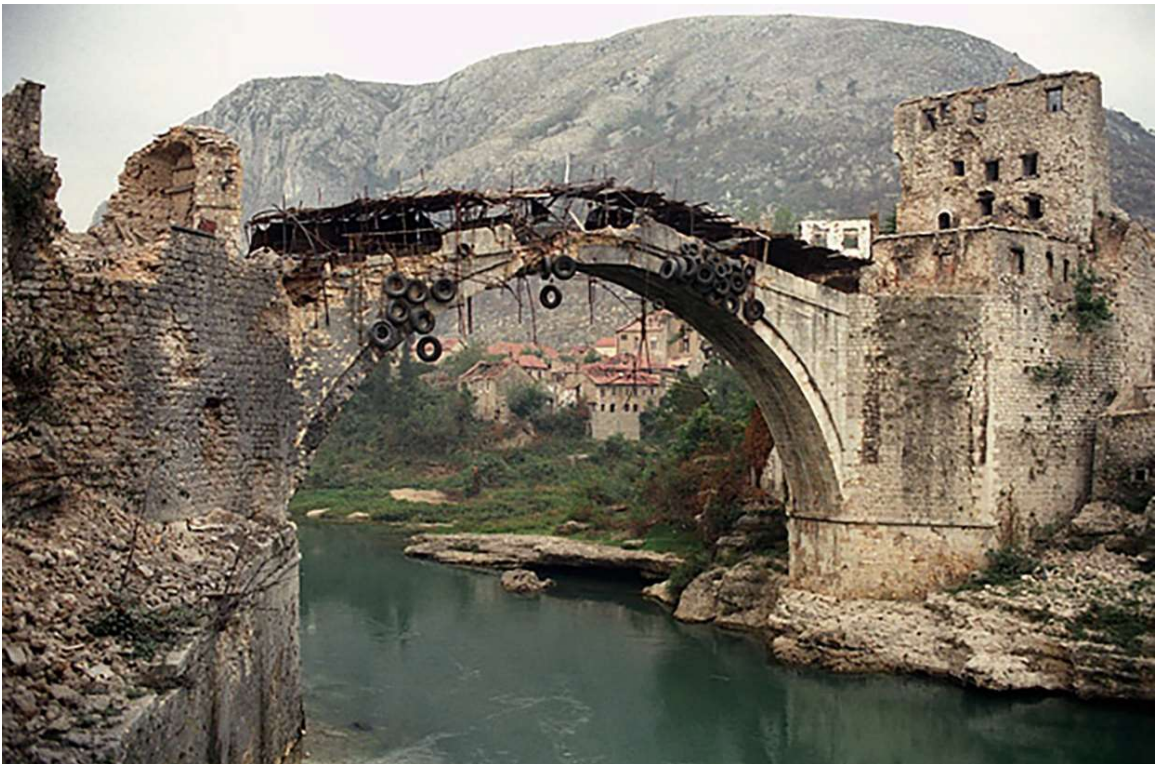
Figure 1. The Old Bridge in Mostar, Bosnia and Herzegovina, destroyed during military operations
